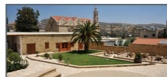
Yermasoyia Cultural Centre Limassol
